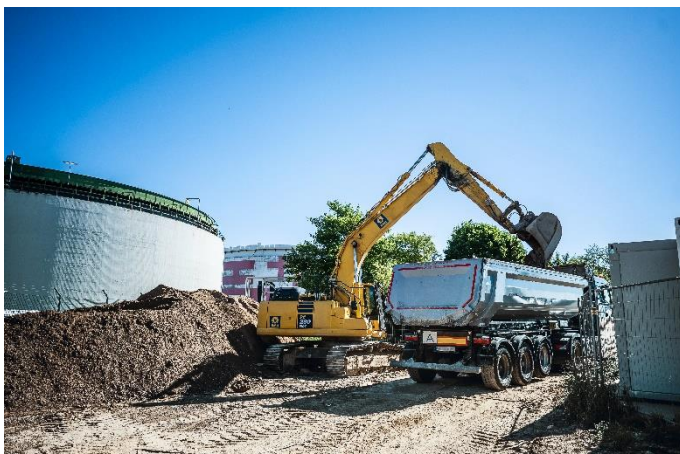
(2) Brownfield remediation and disposal worked hand in hand on this project.
